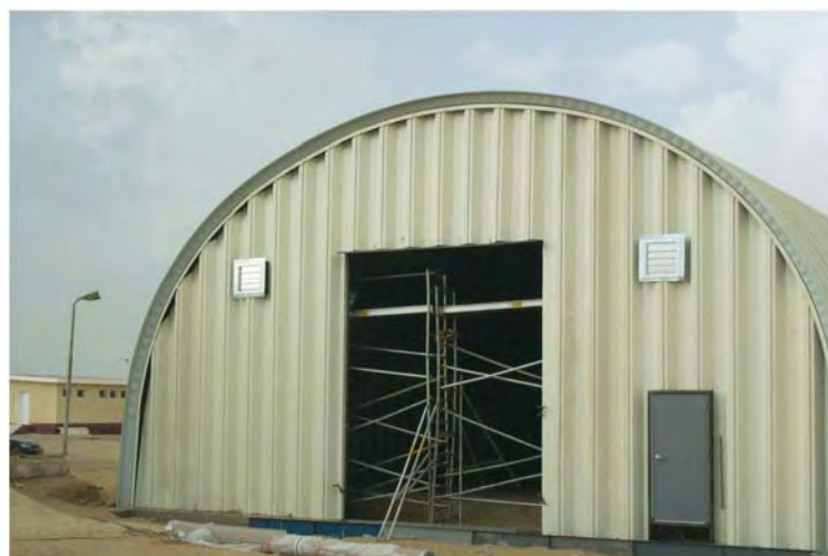
ENDWALL WITH ROLL-UP DOOR INSTALLED
